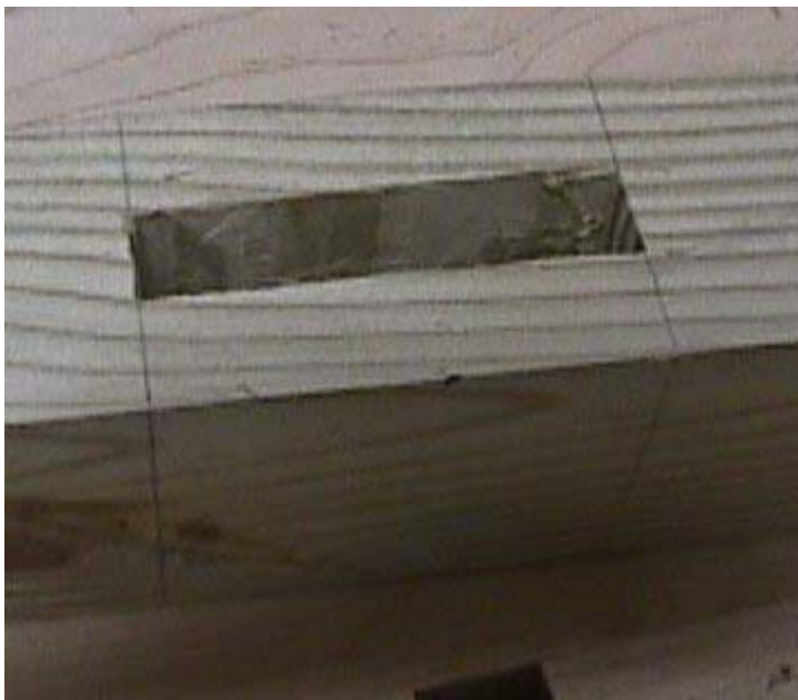
A finished mortise
