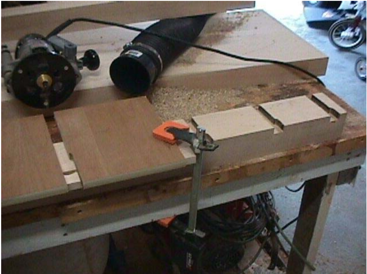
Jig clamped to strip ready to be routed.
