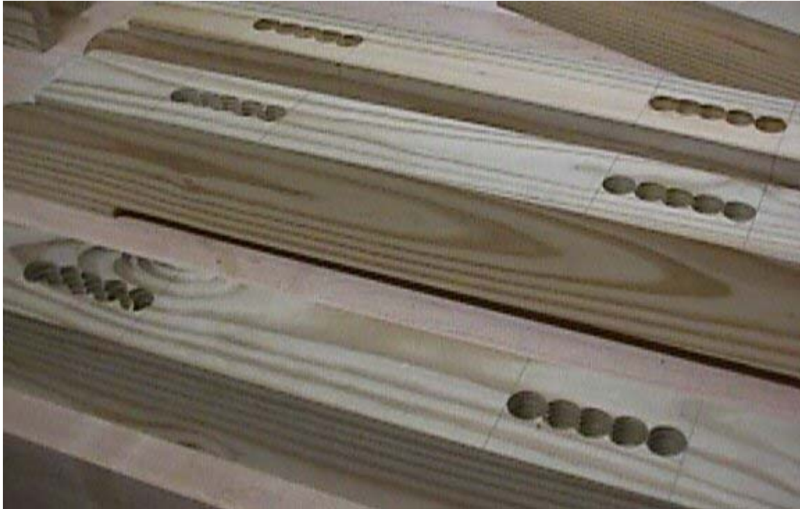
The holes drilled ready for cleaning up into mortises.
